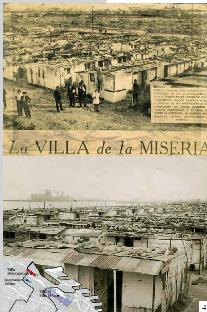
bottom right image, drawing by Rosario Marrocco, 2020). In 1978 one can observe, compared to 1965, the effects of the Plan de Erradicación de Villas de Emergencia conceived by the military government (1976-1983). The inhabitants of Villas 31 and 31 bis go from 24,324 in 1976 to 819 in 1979 and 198 in 1983, then to 7,951 in 1993, 14,584 in 2004 and 26,270 in 2009 (PASTRANA, BELLARDI, DI FRANCESCO 2010: 334).
